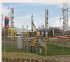
a natural gas power plant
